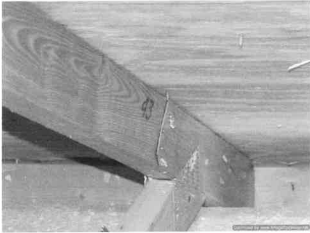
Single wrap with 1 nail min back
